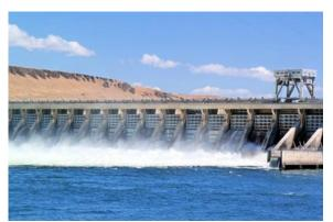
produces electricity. As water flows through an opening, pressure builds up against enormous turbines which causes them to rotate large generators that produce electricity.
